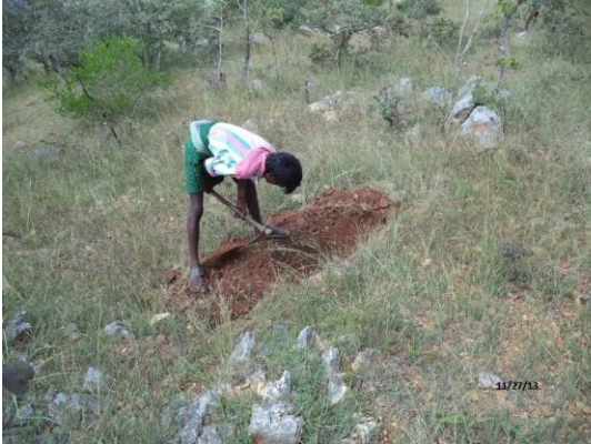
Trenches are 4 feet long & ¾ feet deep and made on hill slopes
