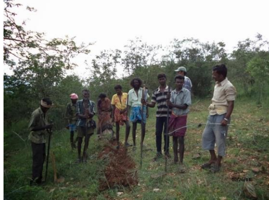
In some places longer trenches of 12 feet have been made
