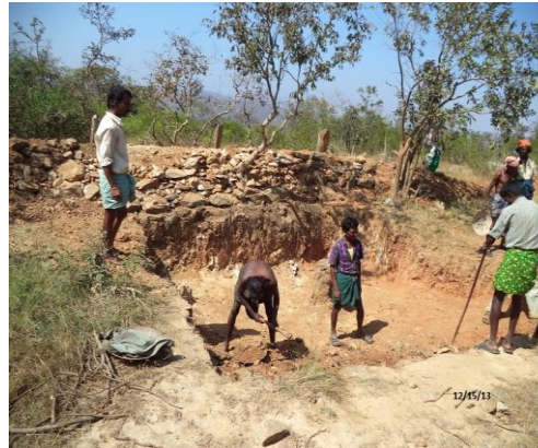
A check-dam type pond digging activity in progress by local community
